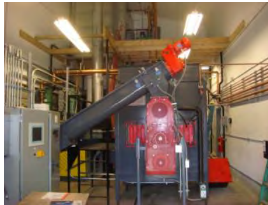
Boiler 3 MMBtuh Hot Water 500 lb/h 25% Char
